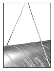
3. Wrap Cable around object being suspended (round duct in this case).
